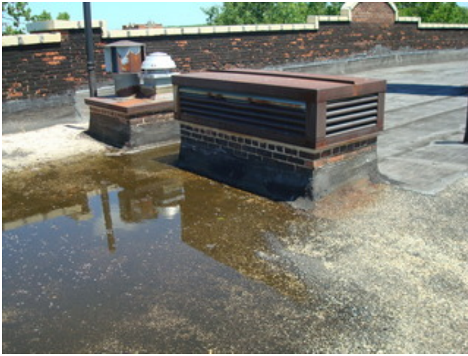
Standing water on Building A 1915 Original Construction
