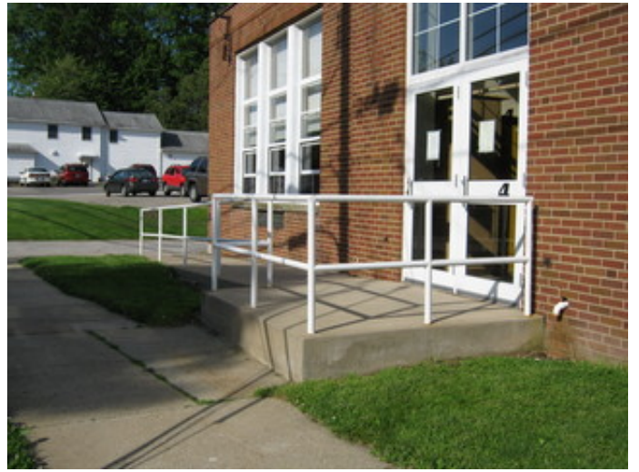
Ramp at building entry
