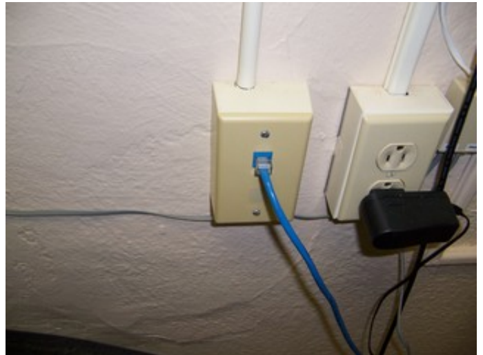
Technology Outlet Site (B)
