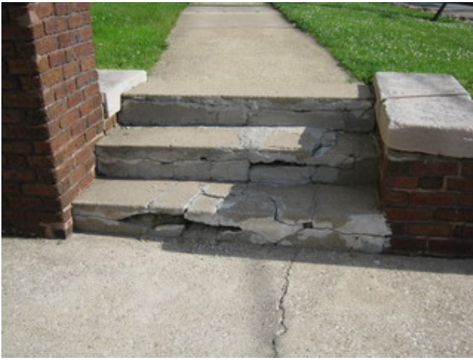
Deteriorated exterior steps
