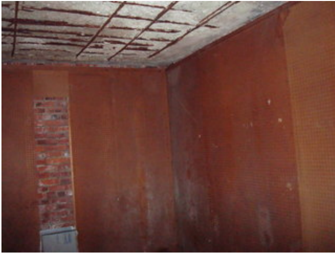
Basement wall in Building A
