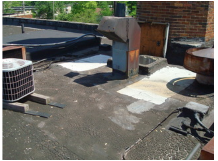
Built-up roof on Building B Original Construction
