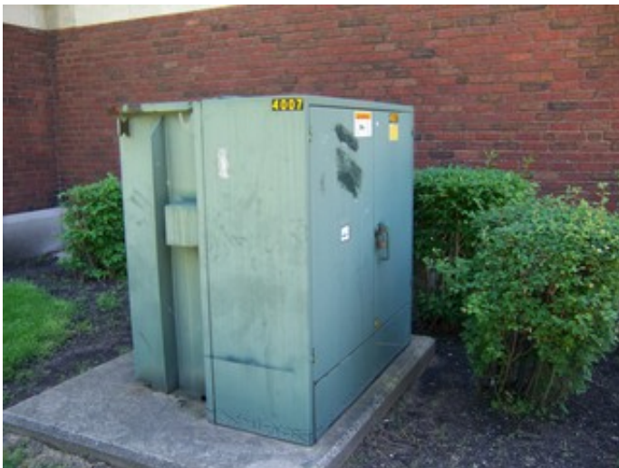
Pad Mounted Transformer Site (A)
