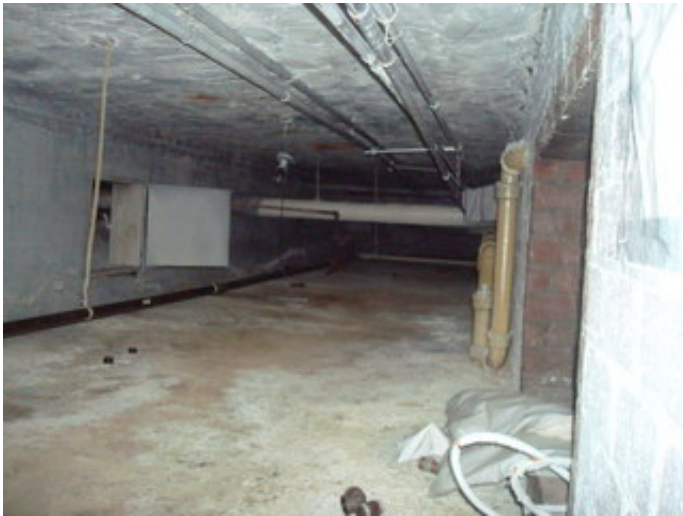
Floor structure in crawl of Building B
