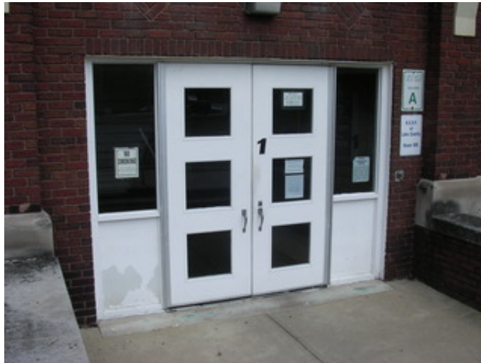
Typical aluminum door Building "A".
