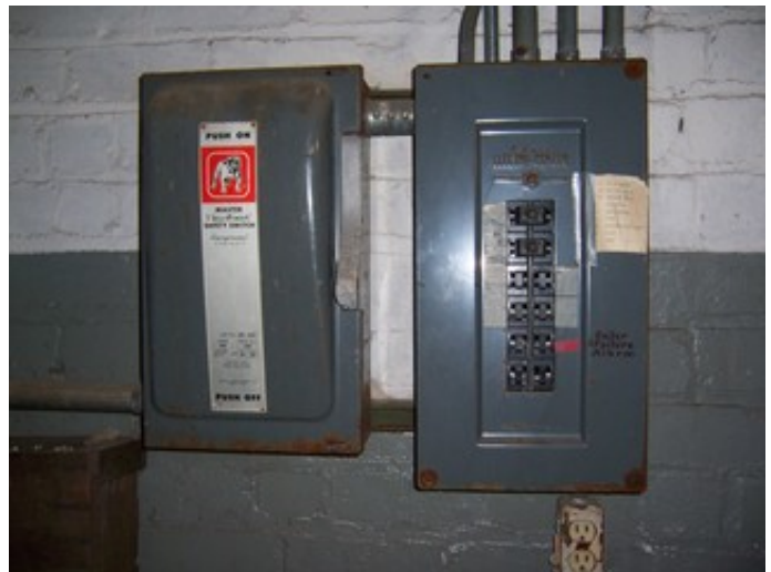
Main Utility Switch & Panel Site (B)
