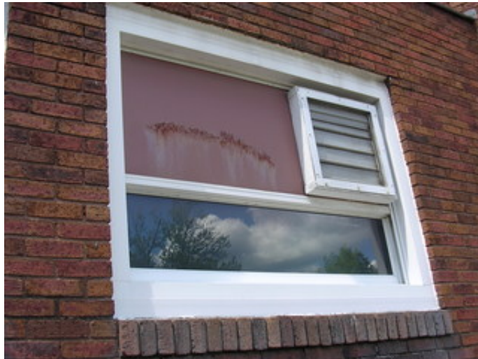
Typical aluminum windows Building "B."
