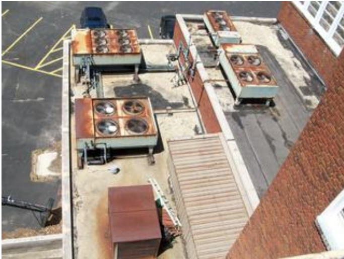
Roof Top Condenser Units
