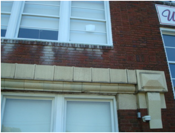
Deteriorated lintel and accent block on 1915 Original Construction to Building A
