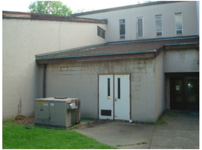
Deteriorated stucco on 1974 Original Construction Building C
