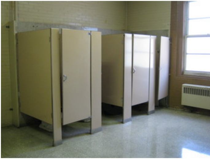
Typical non-compliant toilet partitions
