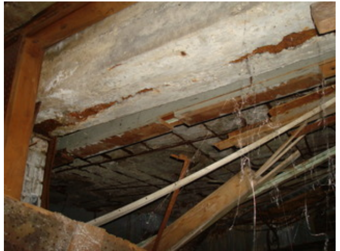
Floor in Building A
