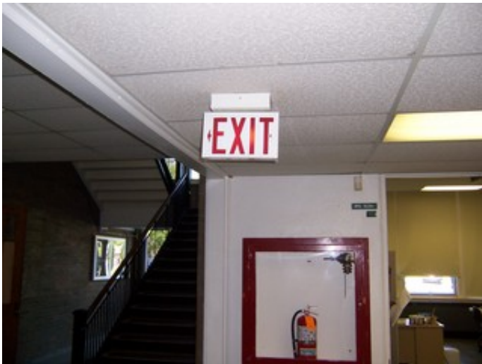
Ceiling Mounted Exit Sign
