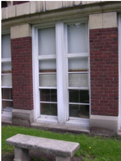
Typical aluminum windows Building "A."
