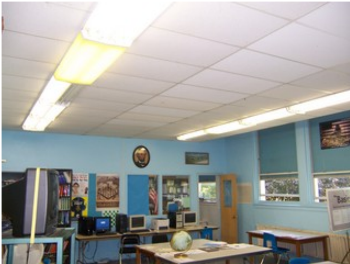
Classroom Lighting Site (B)
