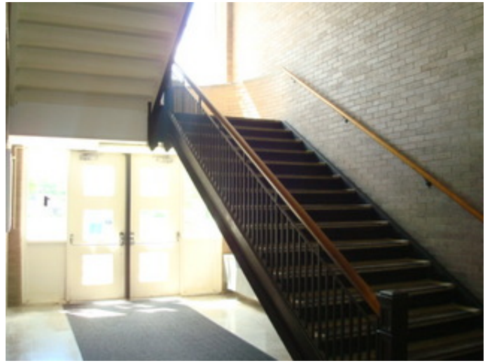
Non complaint stair and handrails
