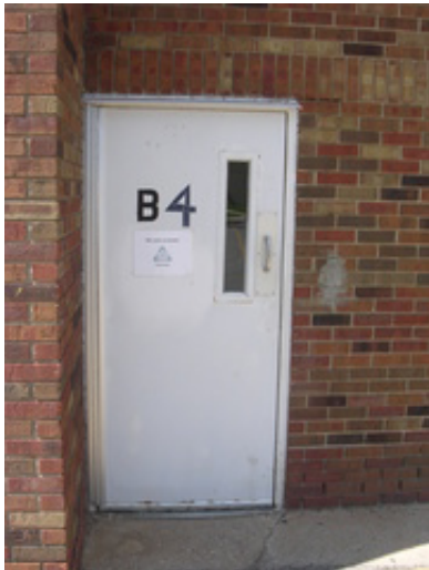
Typical hollow metal door.
