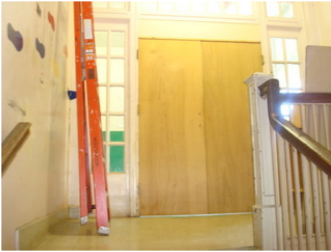
Non compliant door and handrails
