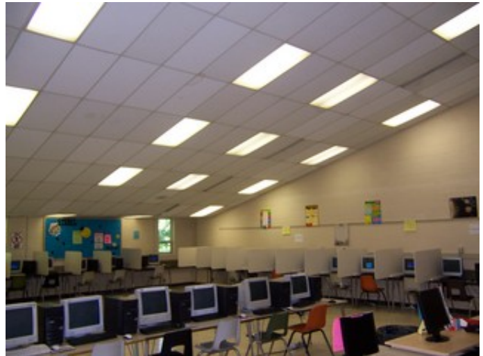
Computer Room Lighting Site (C)
