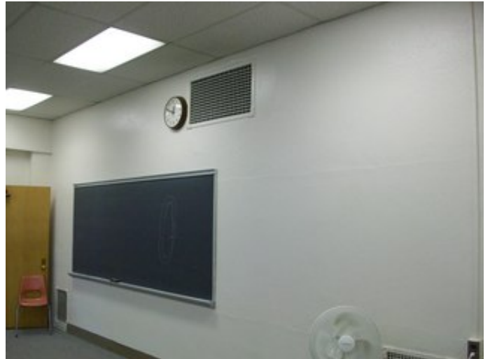
Exhaust Fan/ Roof Venilater
