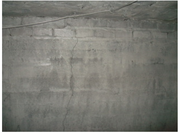
Crawl wall in Building B
