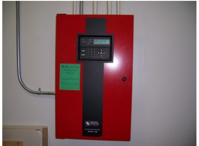
Fire Alarm Panel Site (B)
