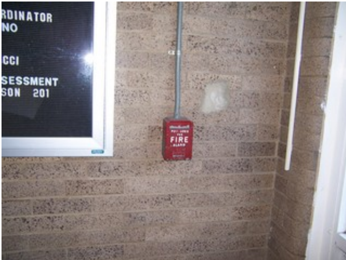
Fire Alarm Pull Device Site (A)
