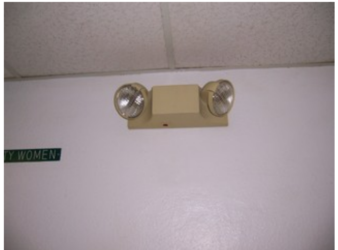
Wall Mounted Emergency Lighting
